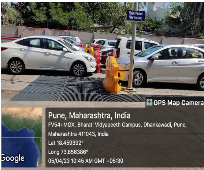
Rain water harvesting
